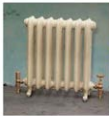
Old cast iron radiators, mainly used in public places
