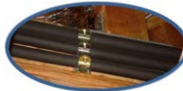
Insulation of support brackets
