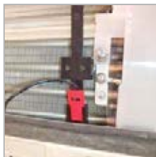
Drain Pan Water Sensor
