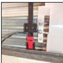
Drain Pan Water Sensor
