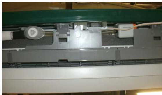
Sample Condensate Pump Example Shown from Below
