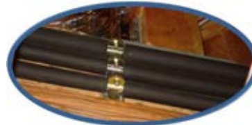
Insulation of support brackets
