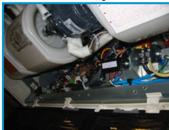
Control and Line voltage connections
