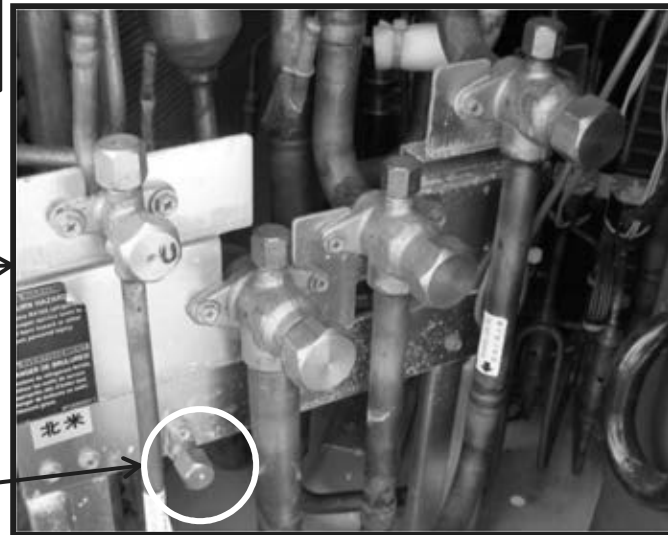
Liquid - Suction-HP/LP-Equalization
