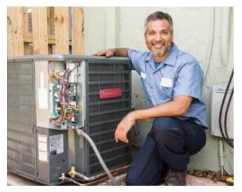
**Compressor** – Converting low-pressure, gaseous refrigerant into a high-temperature gas before it enters the condenser, the compressor plays a critical role in the cooling of your home. The type of compressor is another chief determining factor of a lower or higher efficiency air conditioner. Here are the three most common types of AC compressors:
