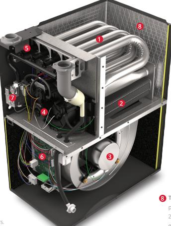
Durable silicon nitride igniter eliminates the need for an energy - wasting pilot light.
