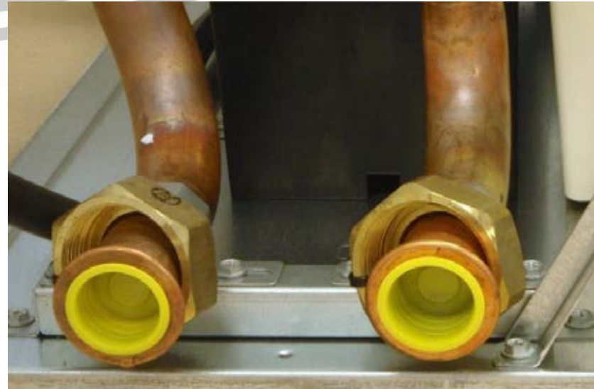
Hydrobox Connections
