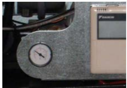
Water Pressure Gauge
