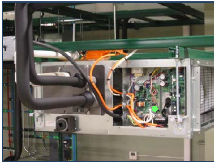
Fan Coil Control PCB
